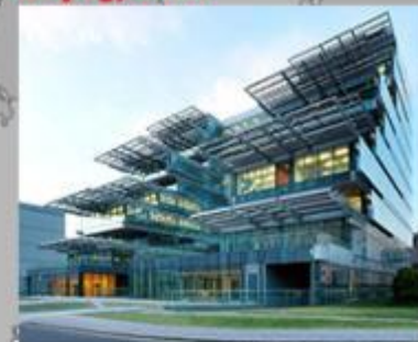
5. Sustainable Building, Tsinghua University, Beijing, China
