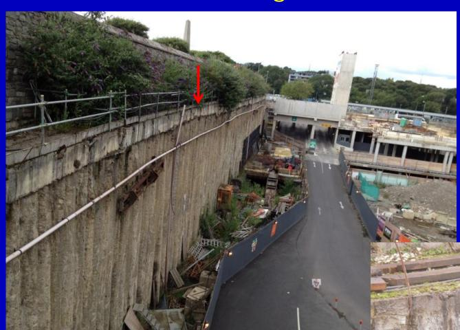
14 m high secant wall with single anchor
