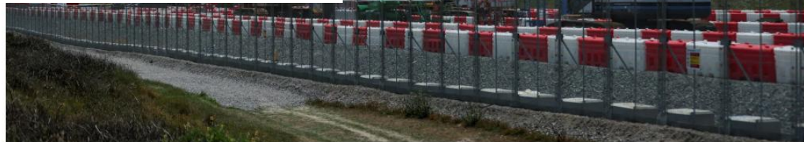
The Sizewell C nuclear power plant construction site. There hasn't been a nuclear plant constructed in the UK for three decades. Credit: Chris Radburn/Reuters
