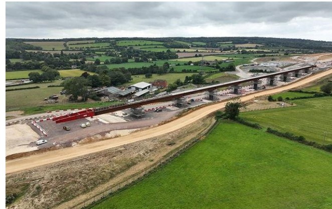
Construction of the Wendover Dean Viaduct, a railway bridge being built for HS2
