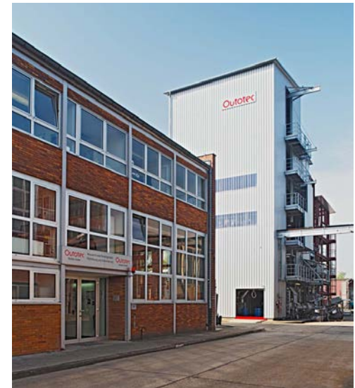
Outotec R&D Center, Frankfurt, Germany.
