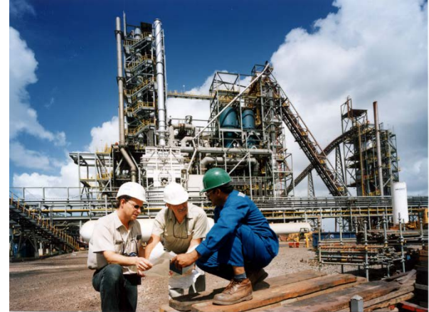
Circored plant Trinidad
