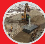
Pre-fabricated steel foundation
