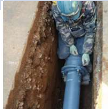
Laying earthquake resistant pipe
