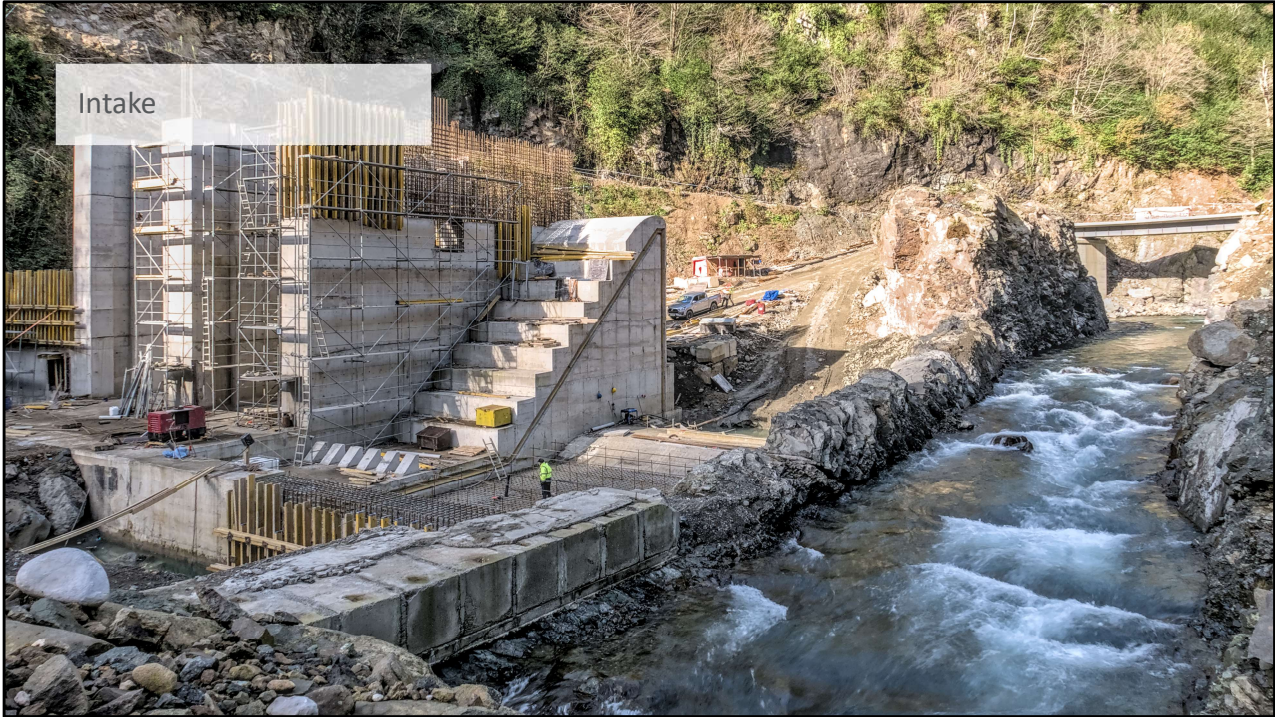
This is a downstream view of the headworks as a reference.*
