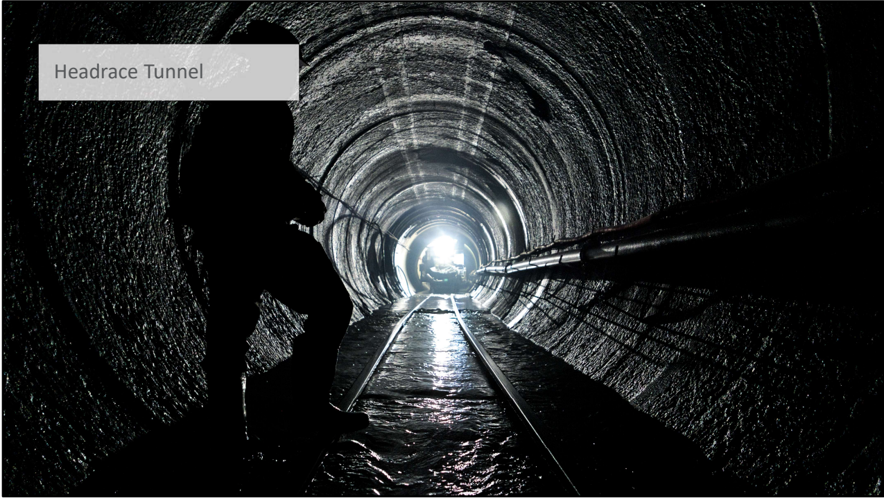
The headrace tunnel, excavated with a TBM and with 3.5 m in diameter.
