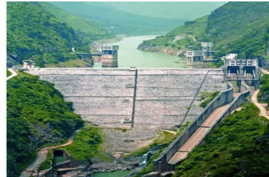
Lubuge Hydropower Project (1982-1990) Rock-fill Dam 101m, 4x150=600MW, 110Mm 3 reservoir
