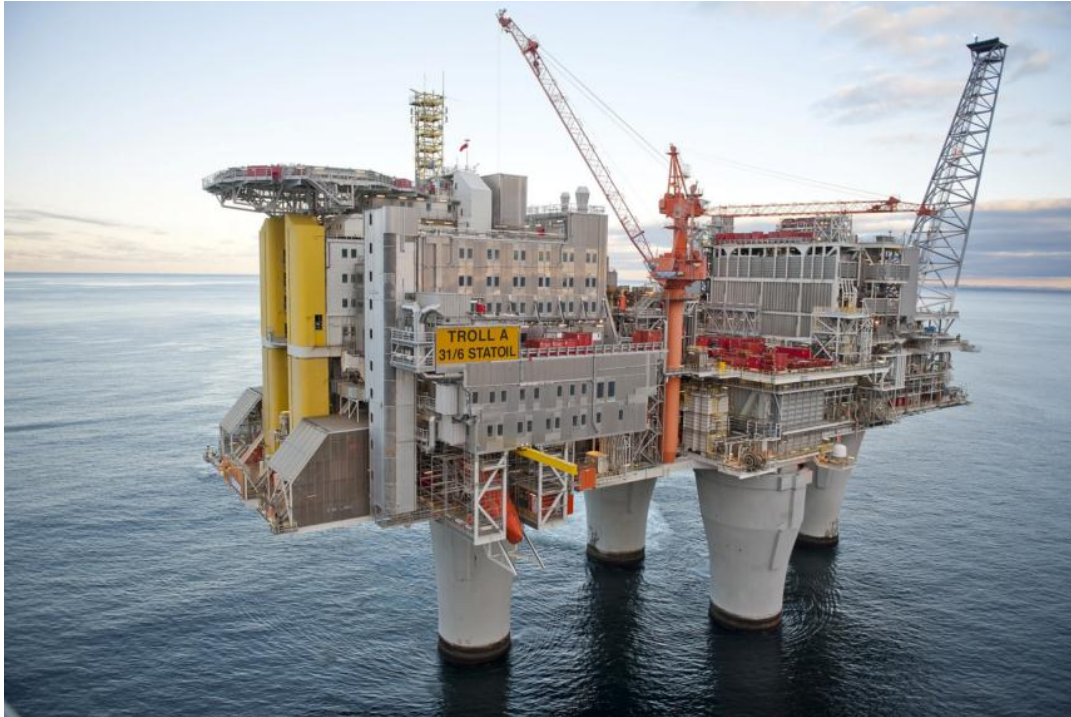
Horizontal drilling has been key to develop the oil reserves at Troll.
