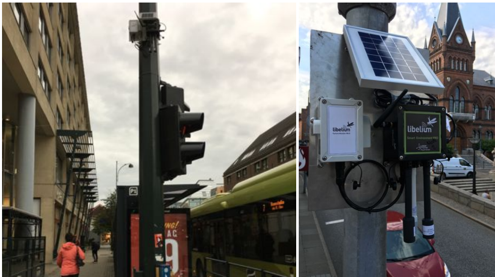
Figure 4 PSSEP deployed in Trondheim (left) and Vejle (right) using deployment plate
