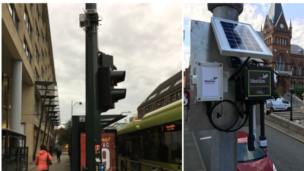
Figure 6 PSSEP deployed in Trondheim (left) and Vejle (right) using deployment plate
