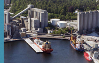
Norcem HeidelbergCement Cement plant
