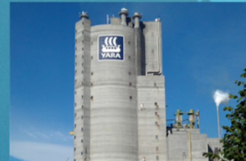
Yara Porsgrunn Ammonia plant
