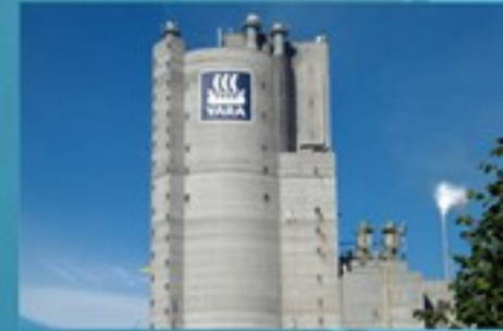
Yara Porsgrunn Ammonia plant
