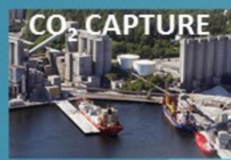
Norcem HeidelbergCement Cement plant
