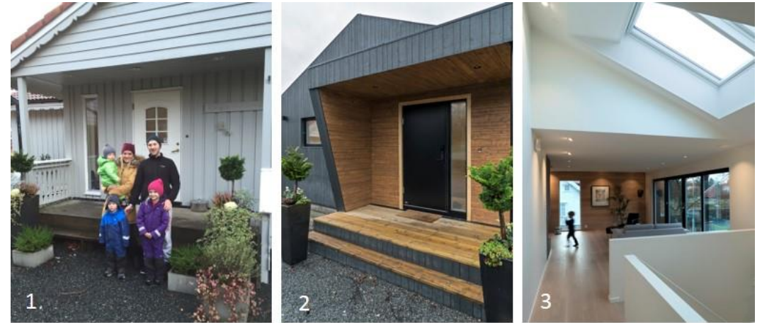
Picture 1: Example from SEOPP, before (1) and after (2 and 3) upgrading. Photo: Jyri Havran.
