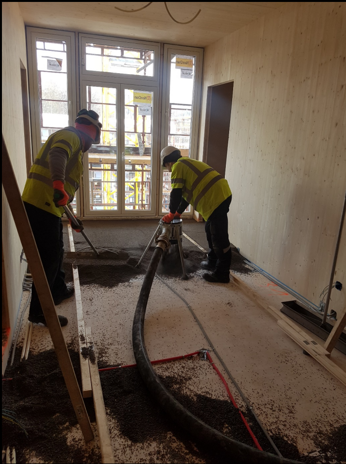
Slabs: CLT, gravels(7 cm) with technical infrastr., acoustic underlay, wood floors, linoleum/vinyl
