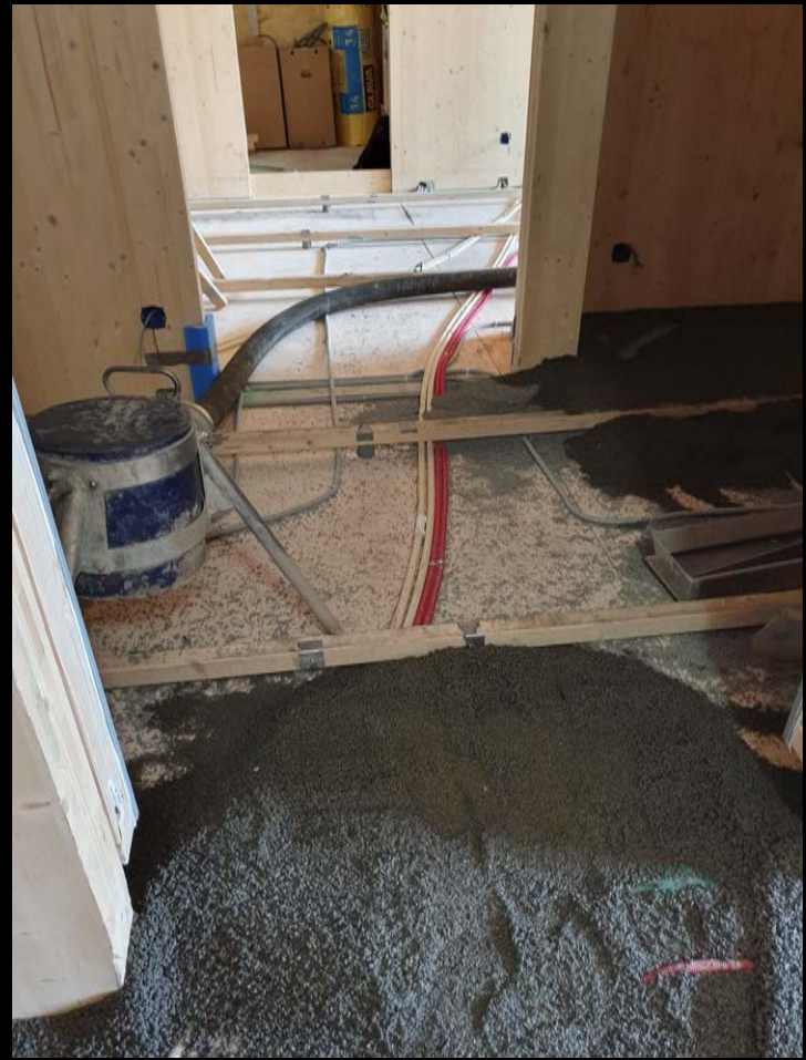
Slabs: CLT, gravels(7 cm) with technical infrastr., acoustic underlay, wood floors, linoleum/vinyl
