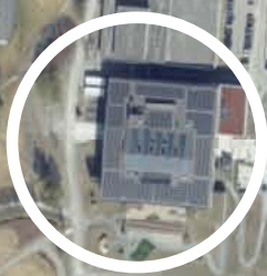
Heimdal high school and sports arena (ZEB-OM)
