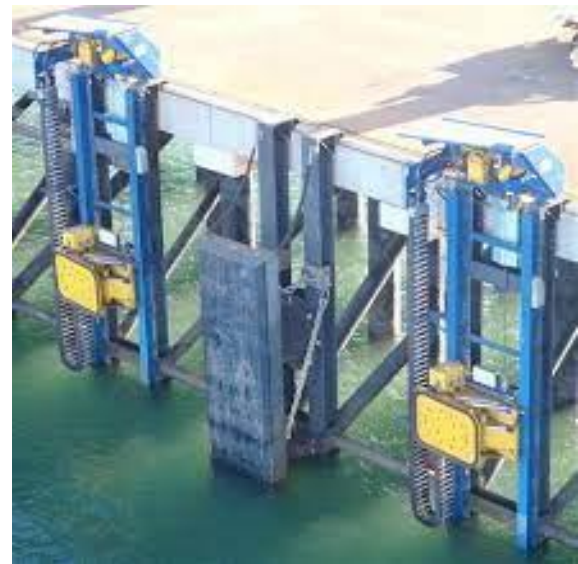
Figure 8: MoorMaster in front of quay. Courtesy: Cavotec.
