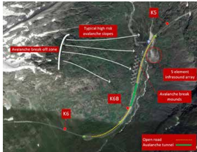
Figure 13. Road stretch at Grasdalen, equipped with FO cable for ~1.1 km length from Grasdalstunnelen (west) to Oppjostunnelen (east). The interrogator unit is deployed in Grasdalstunnelen at K6. The common avalanche break-off zone is on top of the mountain and typical high risk avalanche slopes are indicated with white arrows. Before the avalanches cross the road, most of the energy is supposed to be stopped by the avalanche break mounds. WP4 will analyse detonation released avalanches, potentially self-triggered avalanches and road traffic.
