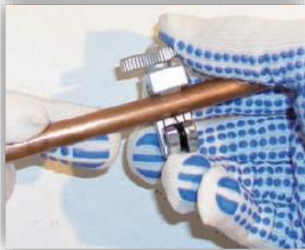
Cutting of Copper Tubes with Tube cutter
