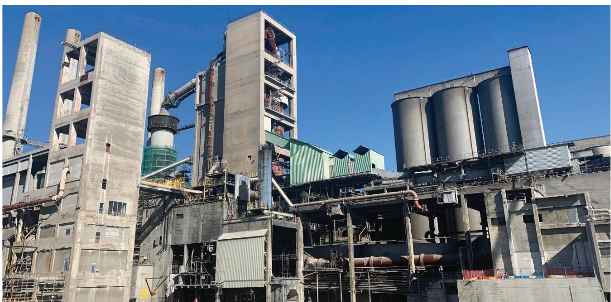
A cement kiln located in Norway, used for the destruction of refrigerant gases.
