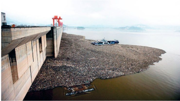
Fig. 1. Accumulation of floating debris behind the Three Gorges (Sânxiá) HPP dam on the Yangtze River, China [4].
