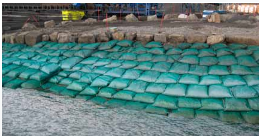
Fig. 42. Erosion protection using geosynthetic containers filled with local soil.
