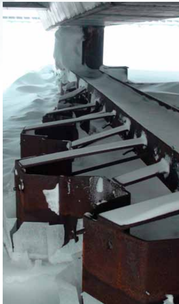
Fig. 6a and b: The deformation of the sheet-pile wall in the main coal harbour at Spitsbergen (Kapp Amsterdam, Svea). Above: a) Local deformation. Below: b) Sketch of ice and water at respectively high and low tides.
