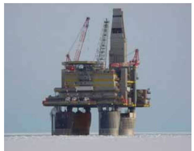
Fig. 29. Illustration of the analogies among different fields. Left: A typical vortex shedding pattern when a flow moves around a cylindrical structure. The oscillating forces interact with the structure, causing it to start oscillating. Right: An ice floe moving around an offshore structure known to give rise to interaction and oscillation of the structure. Could there be some similarity between the two? And what can we learn from the experience in the field of VIV?
