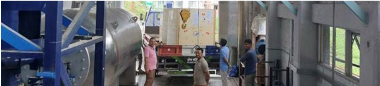
Francis turbine model fabricated in PTM, Norway arrived KU-TTL on August 16, 2024. The installation of the turbine is planned in the presence of manufacturers.
