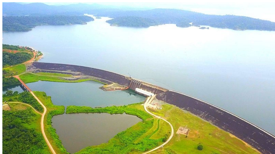
FIGURE 4: AERIAL VIEW OF THE BROKOPONDO DAM AND PART OF THE HUGE ARTIFICIAL LAKE (1,560 KM 2 ) IT CREATED.
