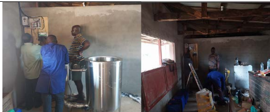
Installation of the electrical components
