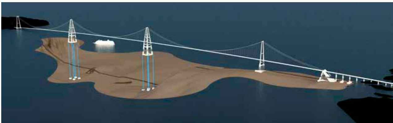
Figure 7: A three span suspension bridge with two floating pylons. Illustration: Arne Jørgen Myhre, Norwegian Public Roads Administration.
