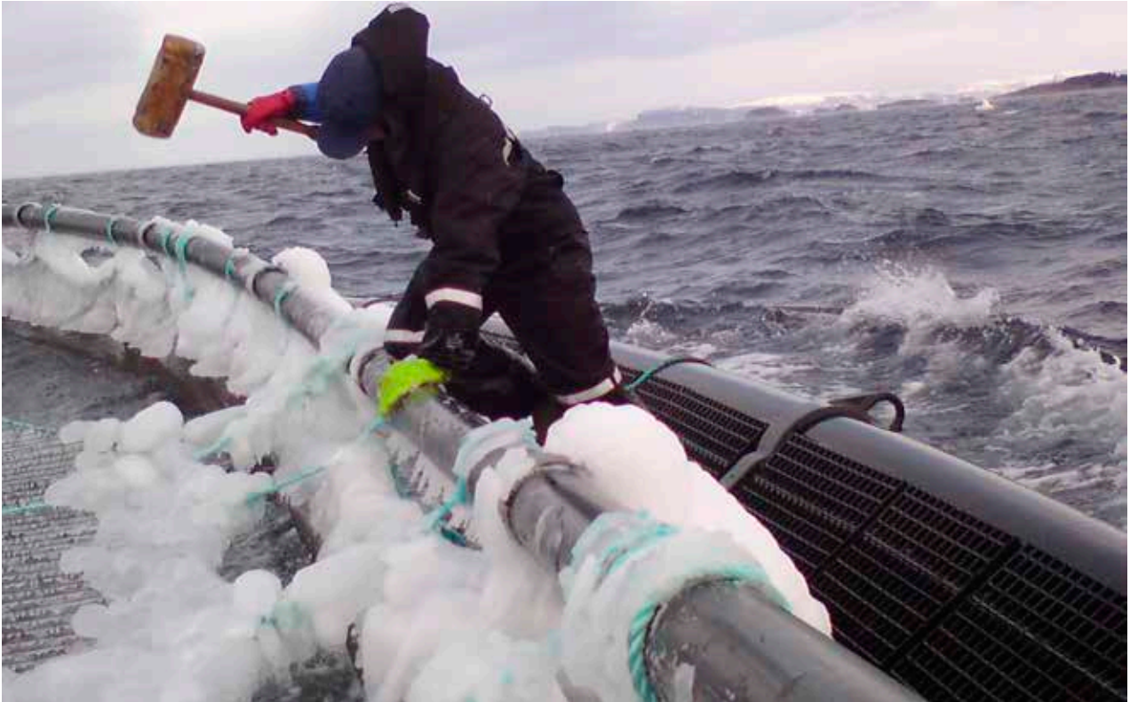
Figure 12: Removal of ice on fish cage. Photo: SINTEF Ocean.
