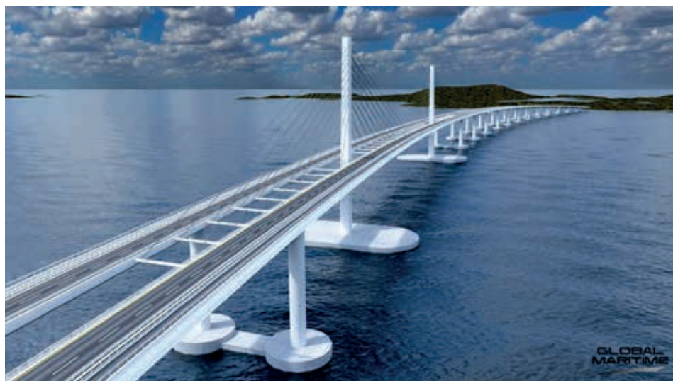
Figure 8:a) Floating cable-stayed bridge in Bjørnefjorden.
