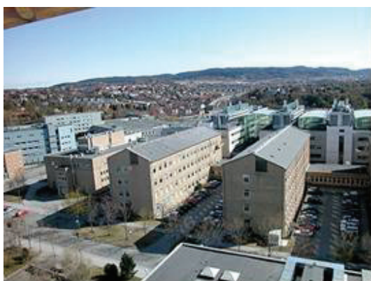
Our buildings, from right: K4, K5, Experimental halls, and the PFI-building (blue)
