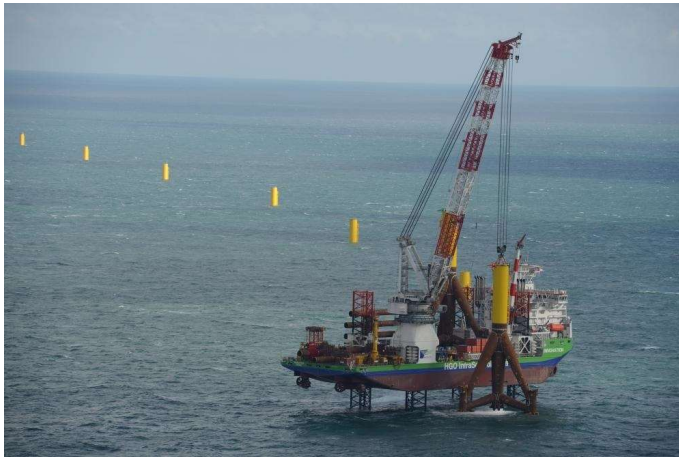
Tripod installation using a jack-up vessel ( http://worldmartimenews.com )
