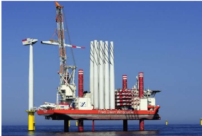
Blade installation using a jack-up vessel ( https://media.licdn.com )
