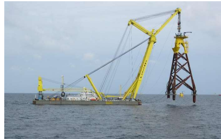
Jacket installation using a floating vessel ( https://www.boskalis.com )
