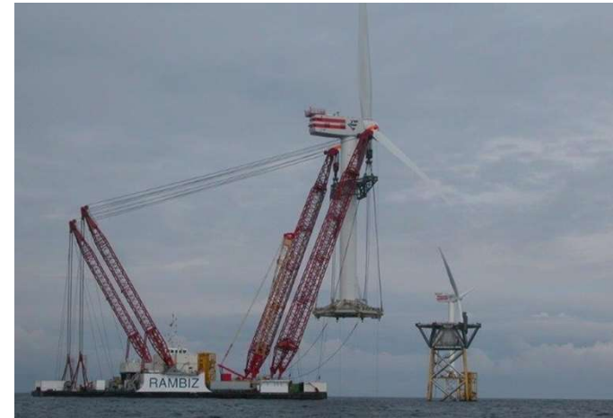
Single lift installation using a floating vessel ( http://www.scaldis-smc.com )
