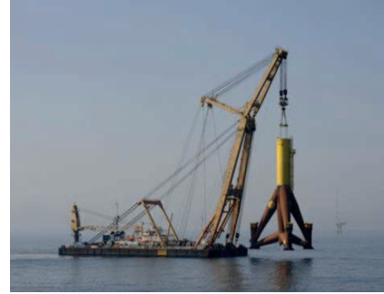
(d) Tripod lifting operation (source: http://www.rechargenews.com )
