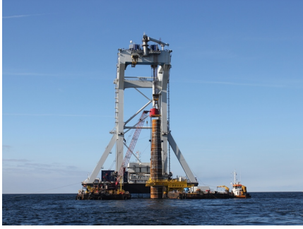
(a) Monopile lifting operation (source: https://www.offshorewind.biz/ )
