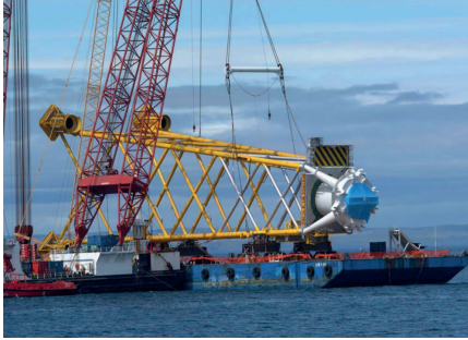
(c) Jacket upending operation (source: http://www.4coffshore.com/ )
