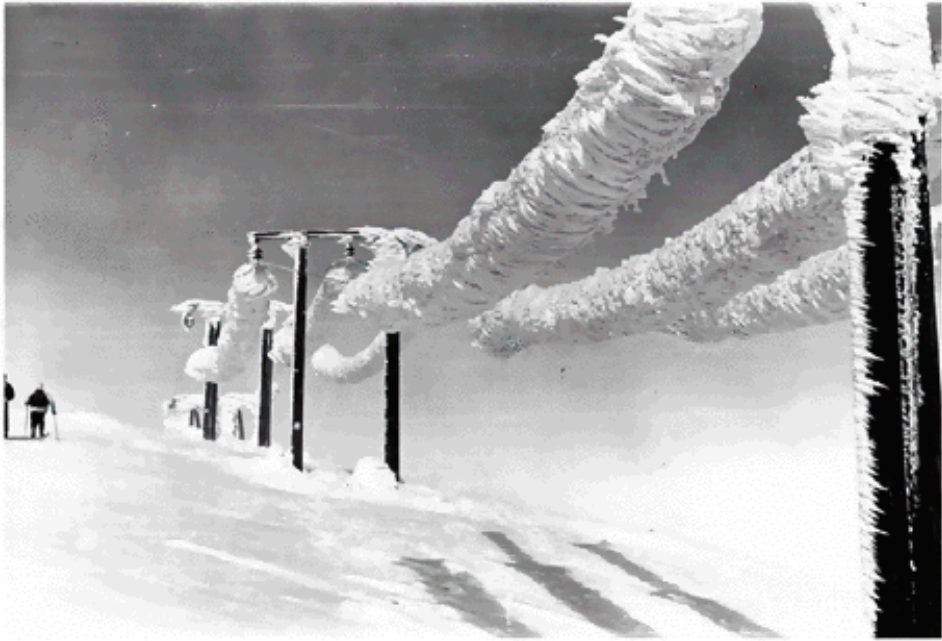
Figure 2.2: Rime icing on a 22kW electric power line in Norway, April 1961, 1400m above sea level. The ice load was measured to 305kg/m [1].
