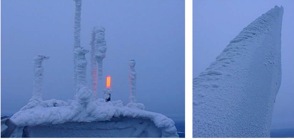
Figure 2.1: Rime ice provoke a temporary de-activation of Äppelbo wind farm (Sweden). Pictures taken from the nacelle, January 2004. Photos: Kjell Jansson, Malungs Elnät AB.
