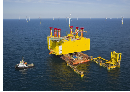
(b) Substation installation using the float-over method. Source: https://www.overdick.com/projects/offshore-wind/hvdc-sylwin_alpha
