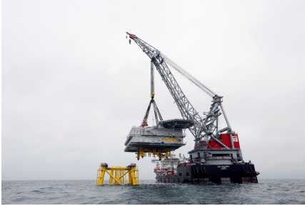
(a) Substation installation using an HLV. Source: http://www.offshorewind.biz
