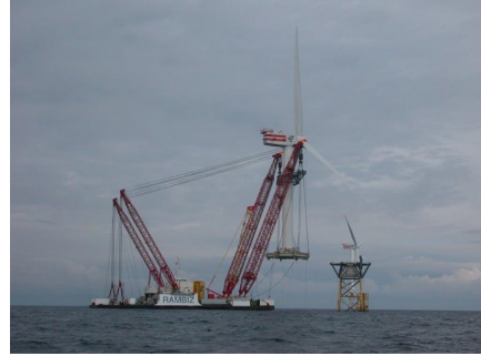
(b) Single lift OWT and RNA installation using a floating HLV. Source: http://www.scaldis-smc.com/en-GB/rambiz-3000/31/
