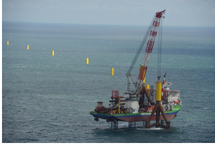
(a) Tripod installation using a jack-up vessel. Source: http://worldmaritimenews.com
