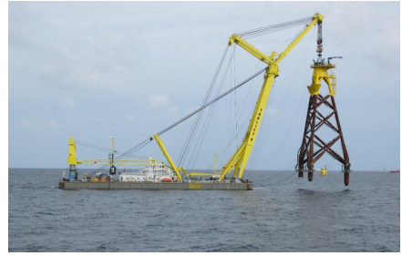
(b) Jacket installation using a floating HLV. Source: https://www.boskalis.com
