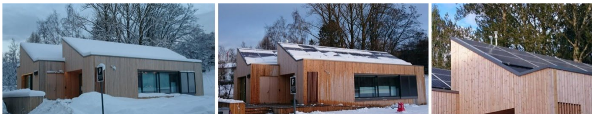
The solar cell panels on the roof of NTNU’s ZEB Living Lab in Trondheim were used as a case study to model how much solar electricity is lost due to snow cover during the winter months.
